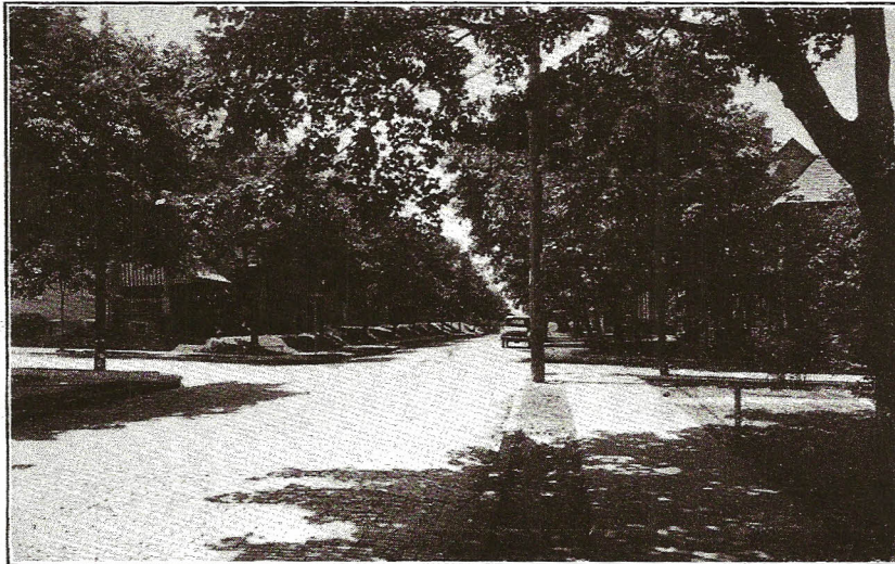
FAIRMONT AVENUE SOUTH FROM FIFTH STREET
